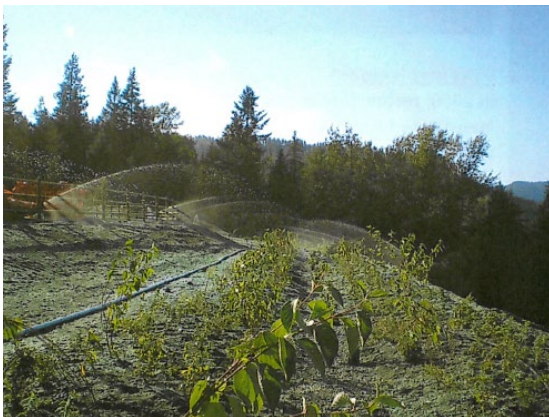
Figure 14: Former Priest River landfill site during remediation.
