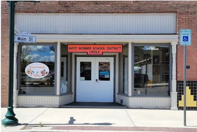
Figure 6: West Bonner County School District administrative office, Priest River, Idaho. Note. Photograph obtained via Google Maps Street View. Photographer and date unknown.
