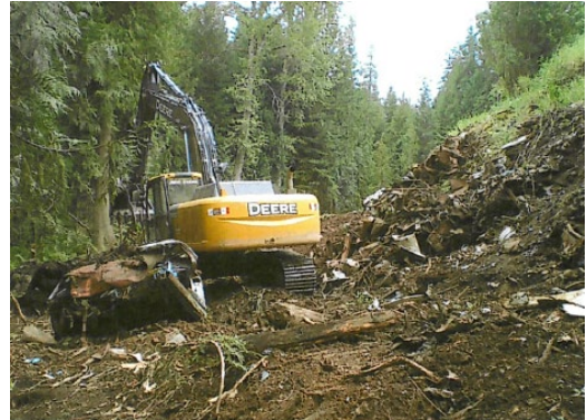
Figure 13: Former Priest River landfill site during remediation.
